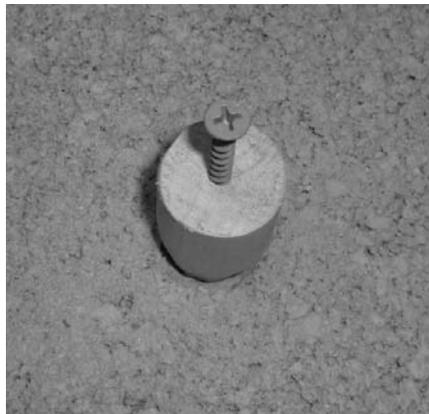
Tighten the screw into the dowel with a screwdriver. Turn the screwdriver clockwise until the screw does not move. Do not over tighten the screw. If the screw is tightened too much, the wall anchor will become unstable.
