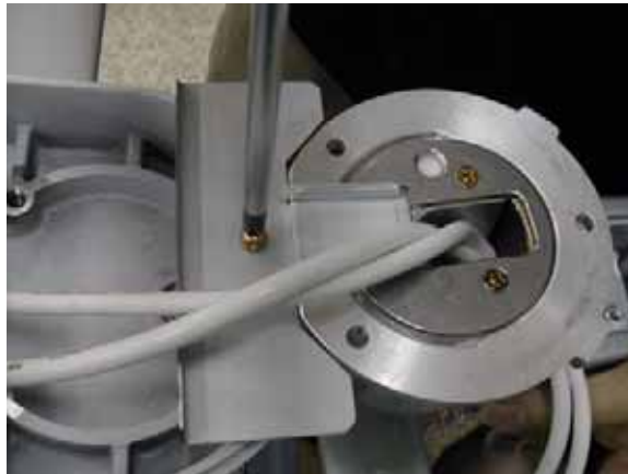
Figure 8-254 Installing OP Bracket
