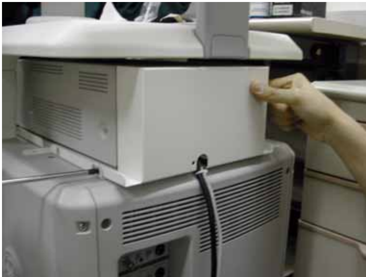
Figure 8-298 Printer VCR DVD Fixture installation top
