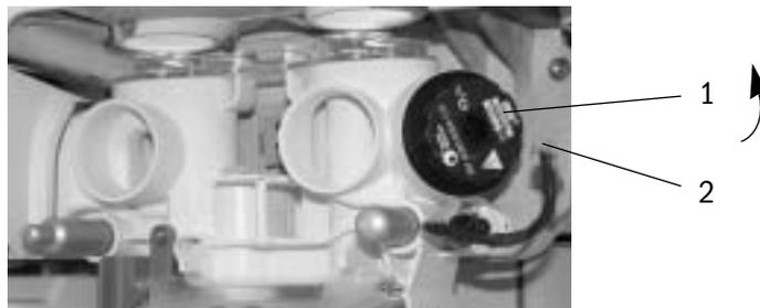
4. Make sure the o-ring (1) is on the sensor. Install the replacement O<sub>2</sub> sensor. Reconnect the O<sub>2</sub> sensor cable.
