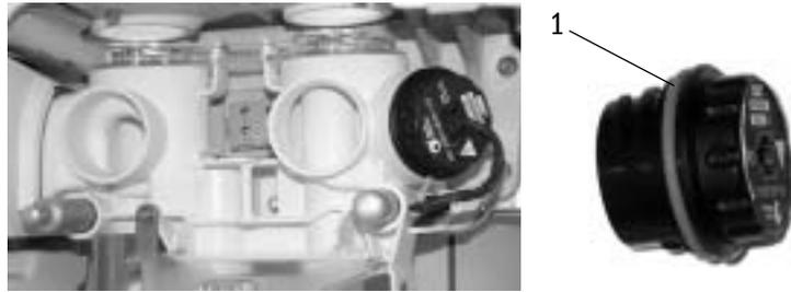
5. Replace the flow sensor module on the system and press the latch (1) in to secure the module.
