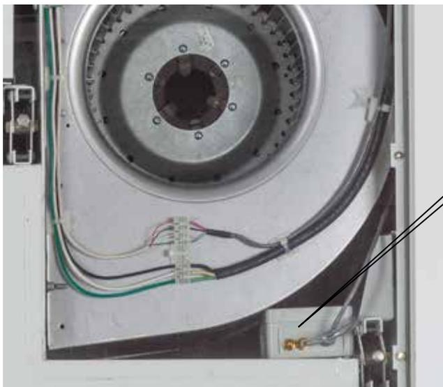
Figure 2.8 Pressure Transducer Location
