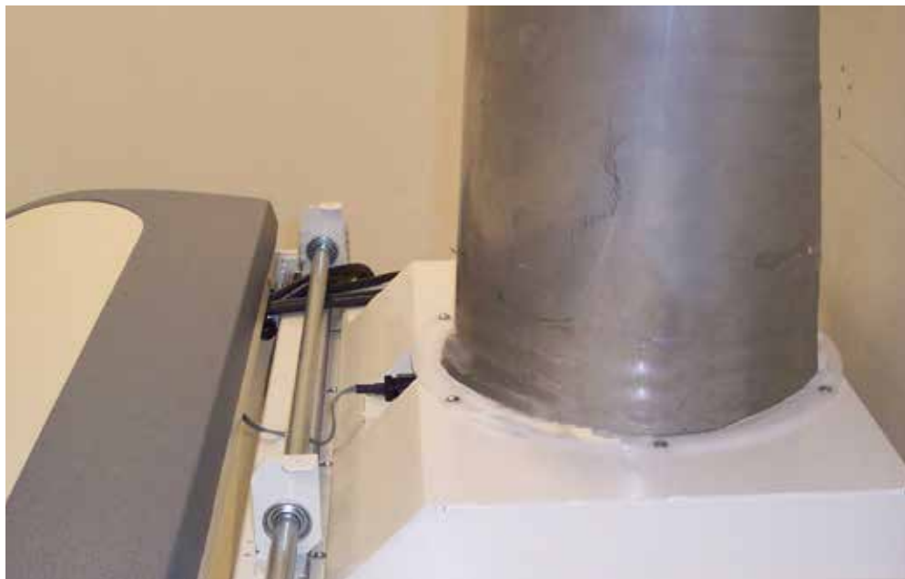
Figure 3.9 Class II B2 Interceptor Duct Connection
