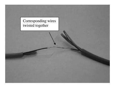
Use heat shrink tubing to provide insulation for each group of wires. Heat shrink a separate piece of tubing over each individual group of wires (see *Electrical-Connections-HeatShrinkTubing*).
