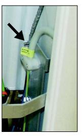
Check whether the grounding straps have complete and firm contact
