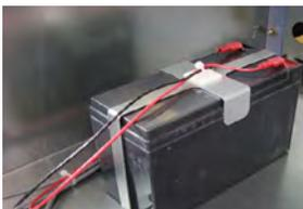
*Monitoring system back-up battery (supplies power to optional Access Control system).*
