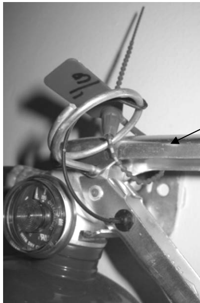
Zip tie securing a safety release pin
