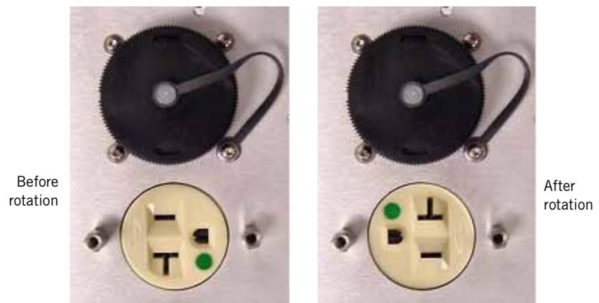
Rotated humidifier outlet allows connection of right angle power cords
