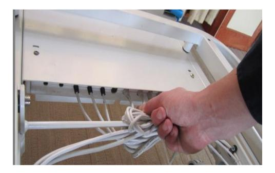
B) Replacing the new control box onto the bed, the procedure is contrary;
